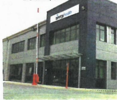
A Synergy off-site SPD facility in Sheffield, UK
