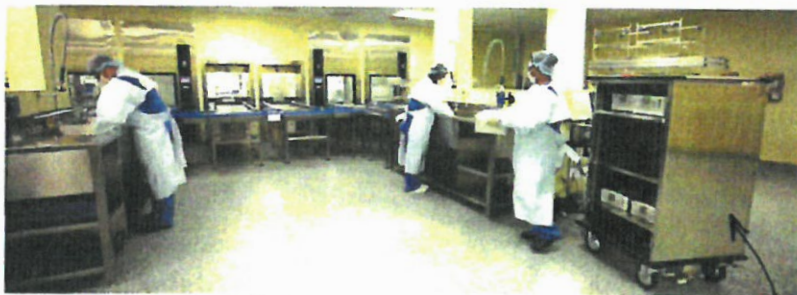
Leesar: Decontamination - in-line sinks and high capacity STERIS Vision washer/decontaminator
